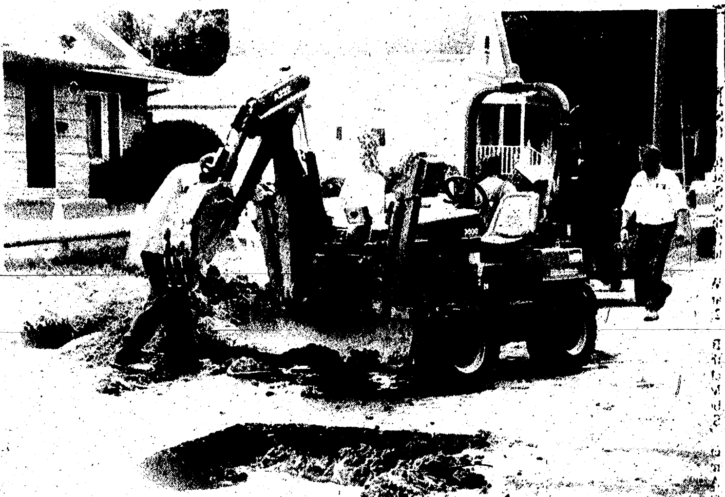
MULTIPLE DISASTERS were reported Monday when MichCon crews ruptured a water main on Dewey St. and when public works crews arrived to repair it and in turn ruptured an old gas main. Gas bubbled through the water and leaked through the pavement until both crews solved their respective problems. Pictured is Dan Rosentreter, superintendent of Chelsea's Department of Public Works, with crews from Michigan Consolidated Gas Company.
